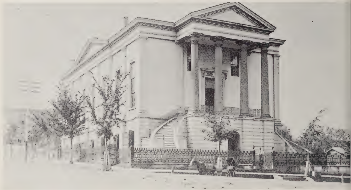
County Court House at the Southwest Corner of Lawrence Street and Washington Avenue completed in 1854 to replace the wooden building on Court Square. A center section and west wing were later added with columns across the center. The iron shutters shown on the first floor above were still in use when the building was demolished in 1958.
